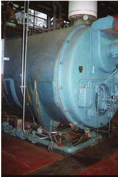
**In addition to these periodic tests of the low water device, the float chamber on the water level control and/or the low water fuel cutoff should be thoroughly flushed to remove any accumulated sediment. At least once a year, water level controls and low water fuel cutoff devices should be disassembled, cleaned and checked.** These devices are an important part of boiler safety. Unless you are thoroughly familiar with them, have an experienced technician perform this type of maintenance.
